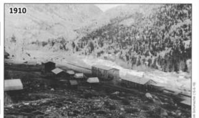
Laramie-Poudre Tunnel Work Site
