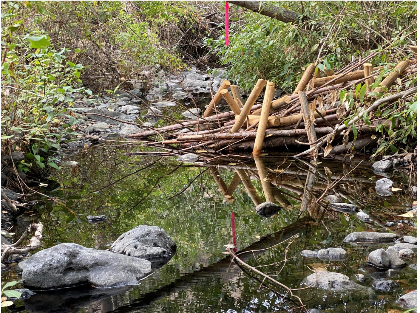
Conservation easement projects for riparian areas are carried out by local partners. Creating artificial beaver dams known as Post-Assisted Log-Structures (PALS) can help retain water in the stream longer, and increase the moisture content of vegetation along streams, potentially reducing the intensity and damage sustained during wildfires. PALS can also be installed post-wildfire in watersheds with a high risk of soil erosion post-fire. Sediment Trap PALS were installed in 2022 in response to the Lick Creek fire and successfully captured fine sediments that would have otherwise impacted water quality in critical salmonid habitat downstream. Photo credit: Asotin County Conservation District.
