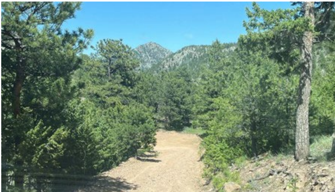
It would not be possible for a firefighting engine to enter this one-lane dirt road in CCCFPD if residents were also evacuating. Photo credit: The Ember Alliance.
