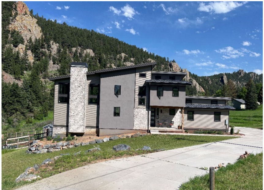
This home in Coal Creek Canyon has many of the recommended home hardening and defensible space measures completed. Photo credit: The Ember Alliance.
