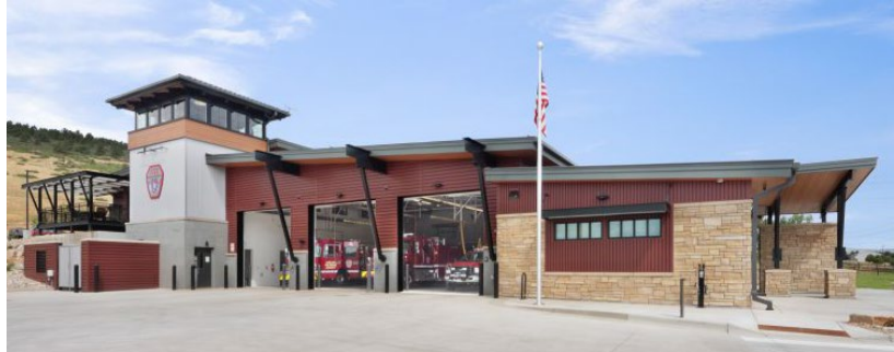
LFRA Station 7, designed with home hardening and defensible space practices. Photo credit: Loveland Fire Rescue Authority.
