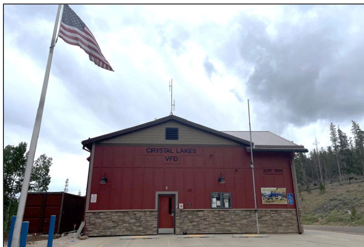
Station 1, headquarters CLFPD. Photo credit: The Ember Alliance.
