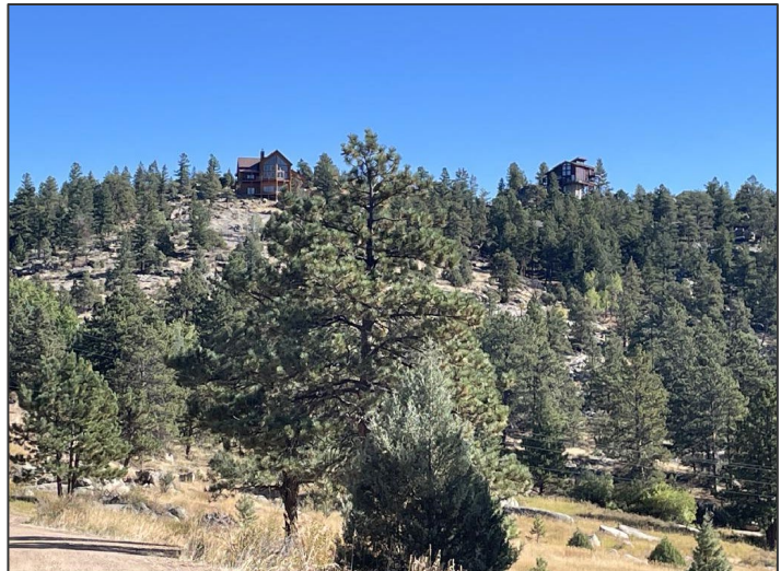
Homes built mid-slope and at the top of steep slopes and within ravines and draws are at greater risk of convective heat from wildfires. A wildfire could rapidly spread up this steep slope and threaten the home above. Photo credit: The Ember Alliance.
